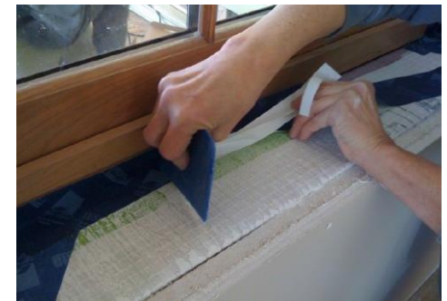
Air tightness. An important but still undervalued aspect of window installation
