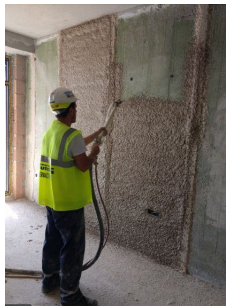
Wet applied insulating plaster
