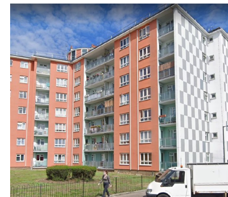
Southwark Park Estate
