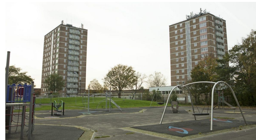
The Channel Island / Exeter Road estate in Enfield has been retrofitted with a communal ground array and individual water heat pumps in each unit.
