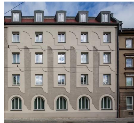
Munich. Housing block renovation.
