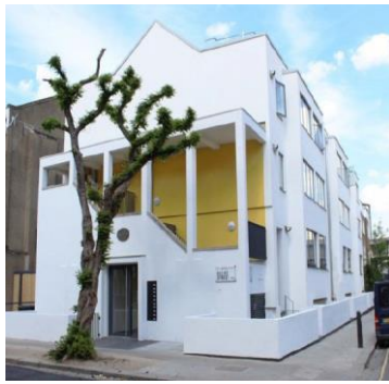
Artic Street, Housing Coop, Camden
