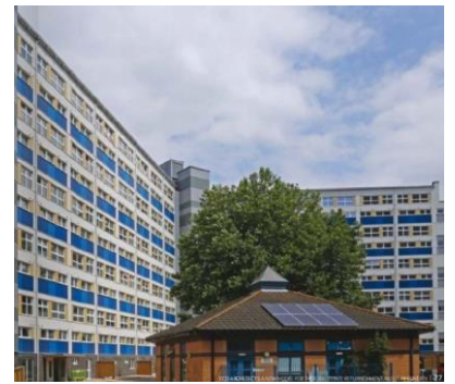
Wilmcote House, Plymouth City Council
